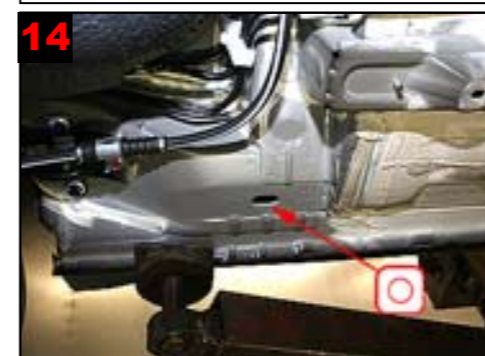
14 Longitudinal member before wheel arch rear: Treat via existing hole.
