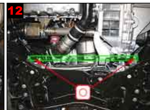
12 Cross member behind engine: Treat via existing holes.
