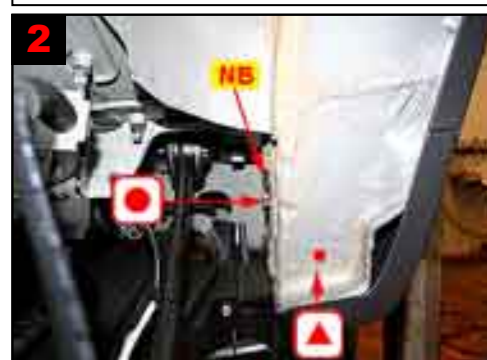
2 Wheel arch rear/panel: Treat via 1 drilled hole and existing plugged hole. NB: Double plating.
